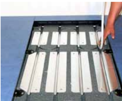
4. Installation of the heating tubes.
